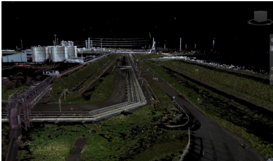
Figure 5 Image from 3D Laser Survey looking at the Overhead Lines from Dabholm Gut
