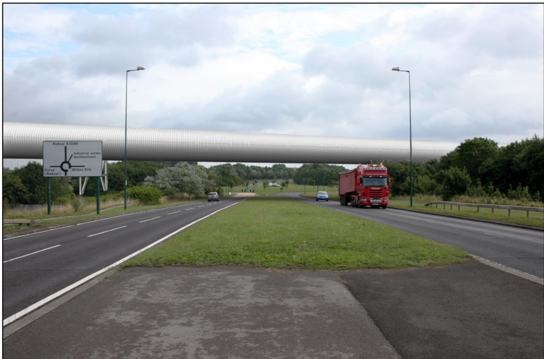
Figure A3.18 D1 - Conveyor only viewed from bridge towards roundabout.
