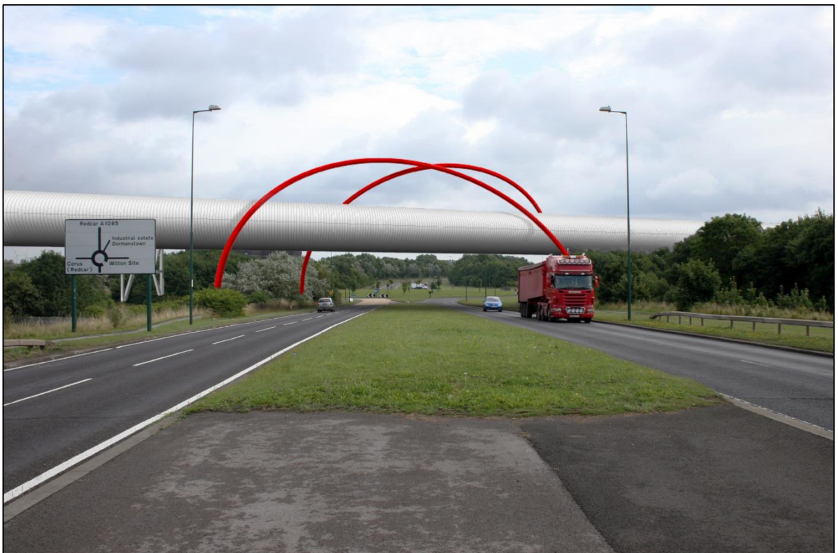
Figure A3.20 D2 - Conveyor and slanted arches viewed from bridge towards roundabout
