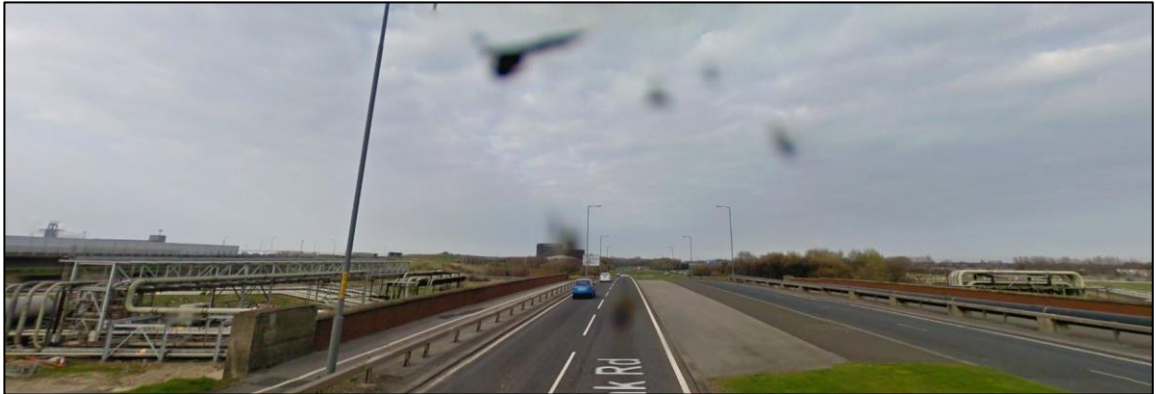
Figure A3.1 Lord McGowan Bridge looking towards roundabout and Redcar beyond.
